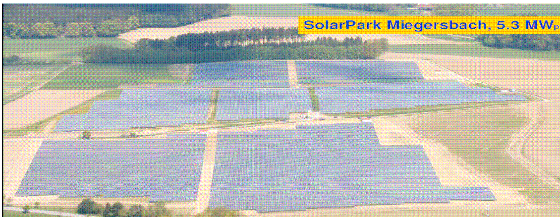
PV-power generation plant
