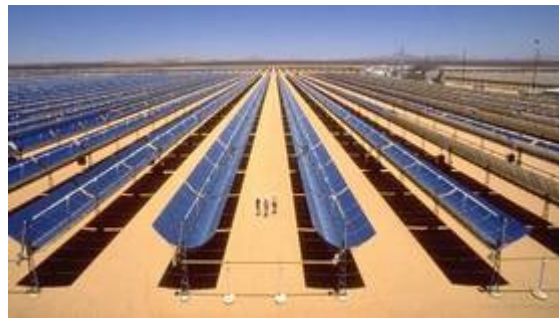
SEGS 350 MW, California
