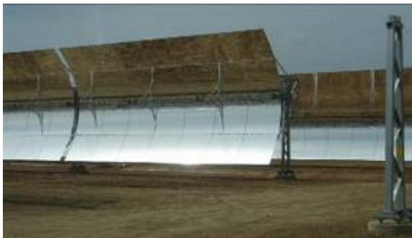
Andasol 2 x 50 MW, Guadix
