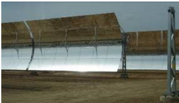
Andasol 2 x 50 MW, Guadix
