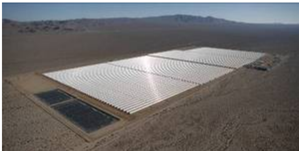
Nevada Solar I, 64 MW
