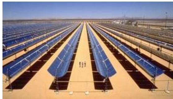
SEGS 350 MW, California
